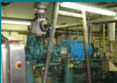
The compressor used to compress the ammonia gas during the chilling process.
